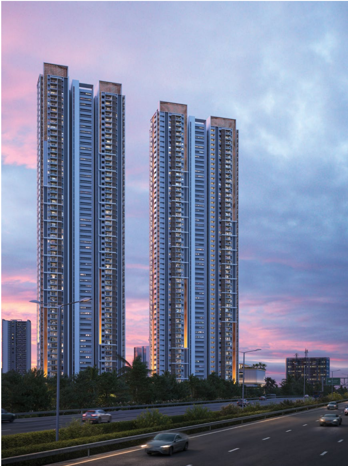
Jayabheri, The Pinnacle at Kokapet, Hyderabad
