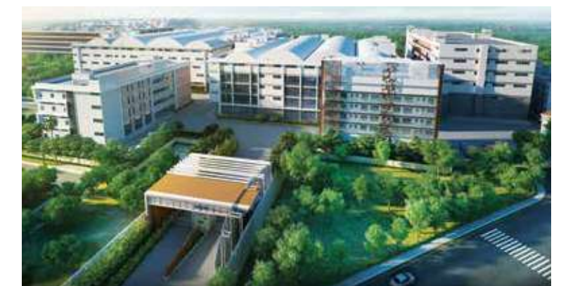
SRIJAN INDUSTRIAL LOGISTIC PARK on NH 6
